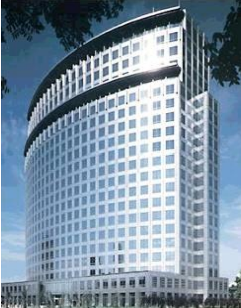
Plaza Tower, Costa Mesa, USA
